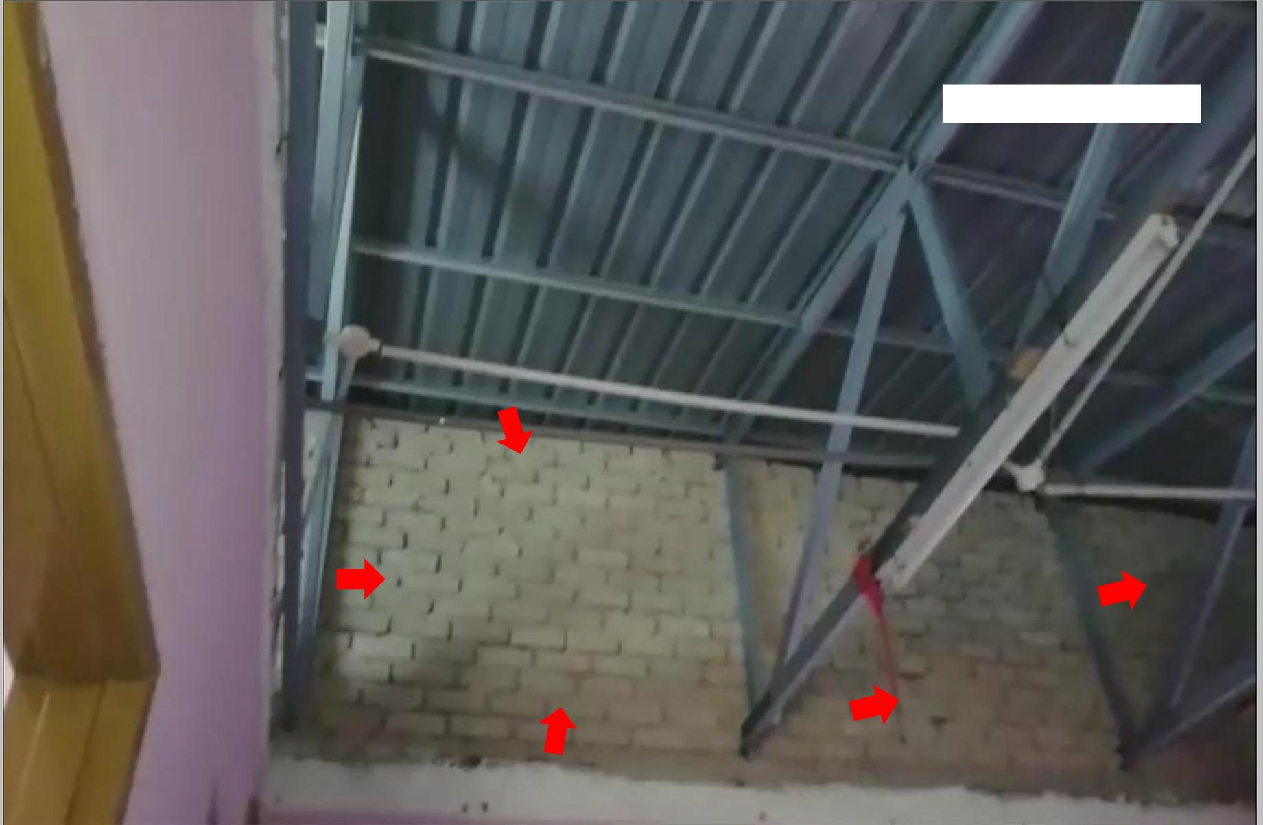
2. Conquas or Q-Lassic should be carried-out upon the completion of the superstructure works ( frame & wall ) instead of upon completion of finishing work
