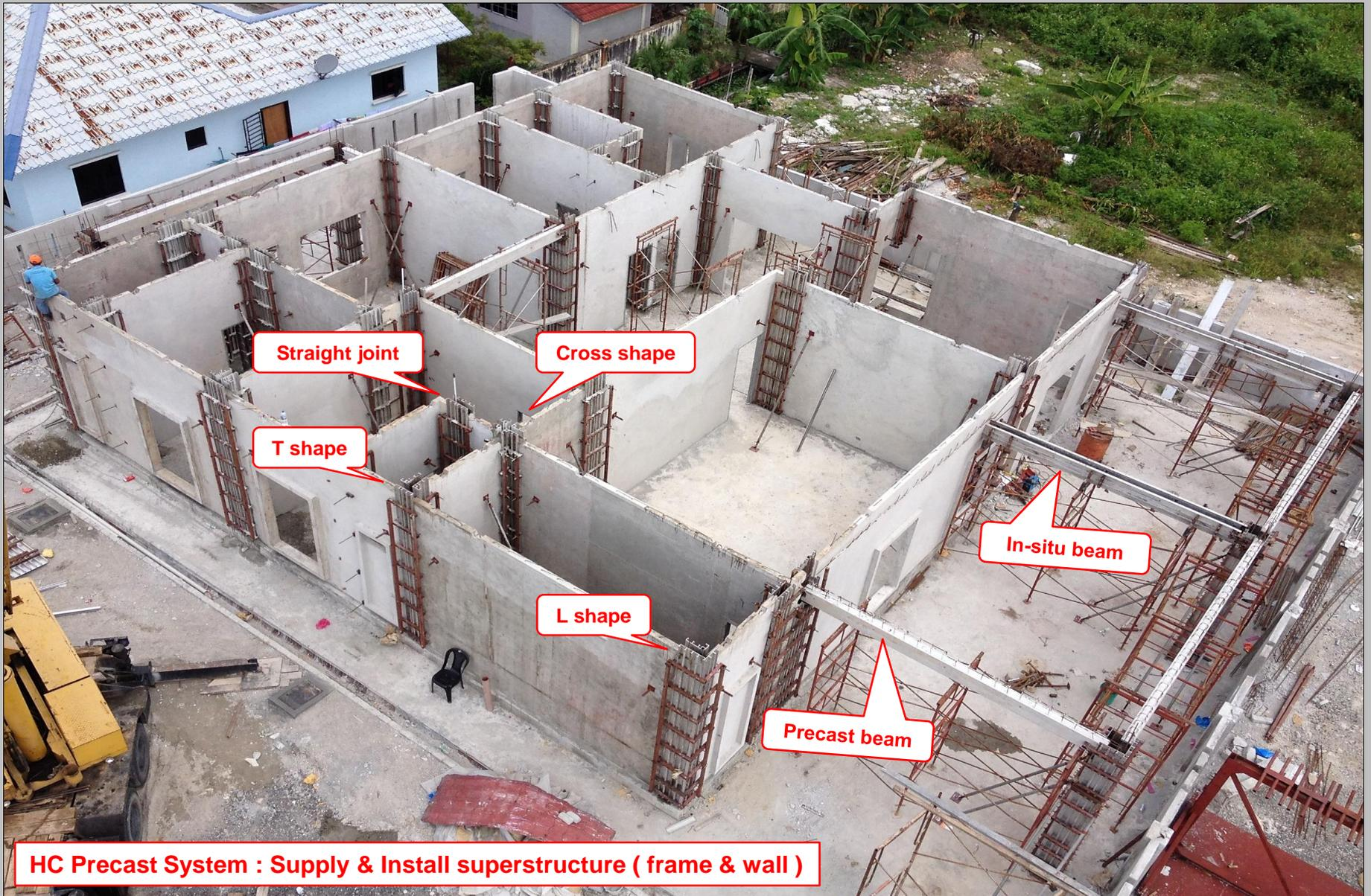
**HC Precast System : Supply & Install superstructure ( frame & wall )**
